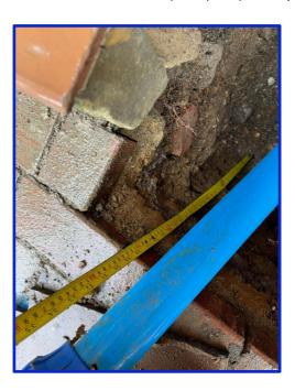
Barrier Pipe approved by British standards (BS 8588) Identified by the black/brown stripes along the length of the outer layer of plastic.
