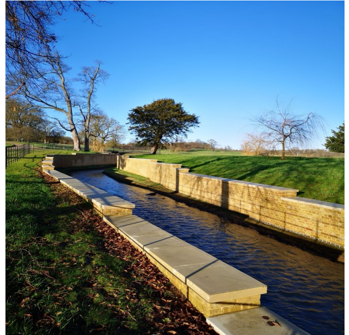
New river channel (pinch point), River Beane
