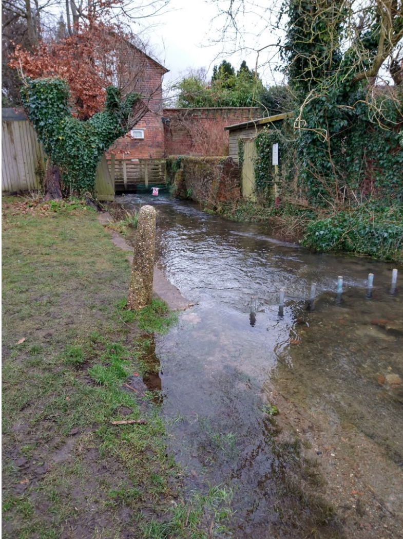
Before - channel during medium-high flows
